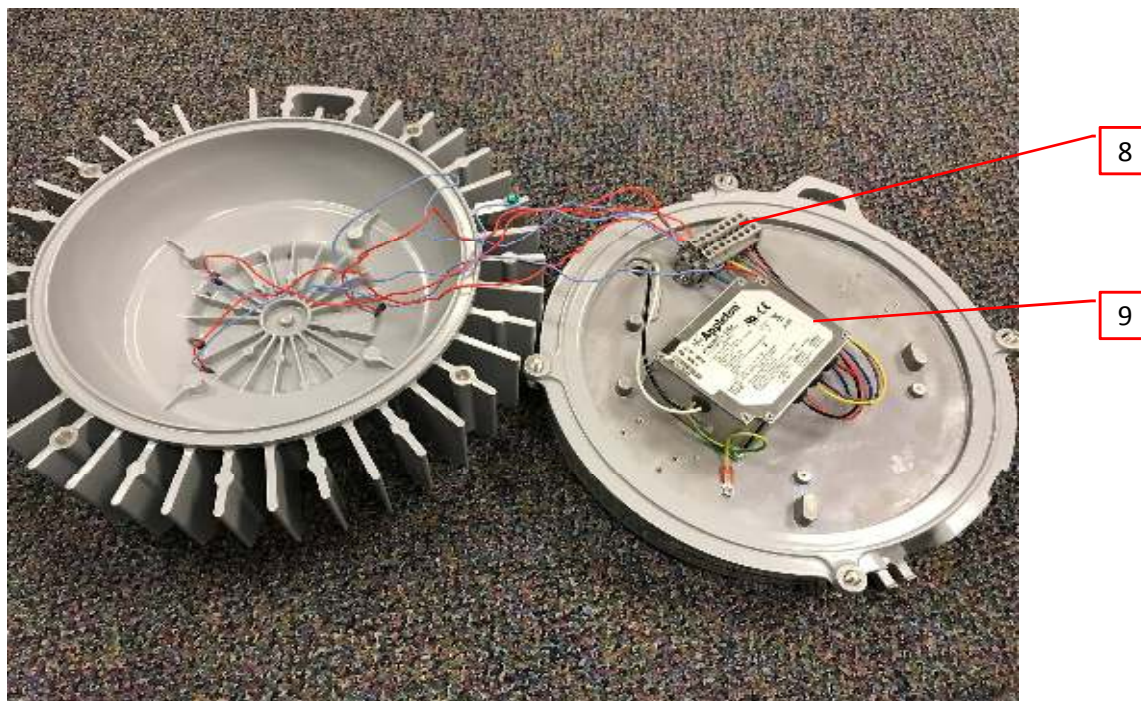
Photo 4 - Internal view of Mercmaster Generation 3 LED luminaire main compartment
