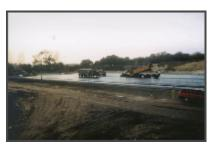
Normally linings in hydraulic works are applied on a drainage layer, capable of conducting any possible seepage in a manner that does not endanger the structure. Such layers need to remain serviceable. In landfill constructions such a drainage system under the lining is undesirable because any localised cracks could be transformed into major failures through the cross-distribution of aggressive substances.
